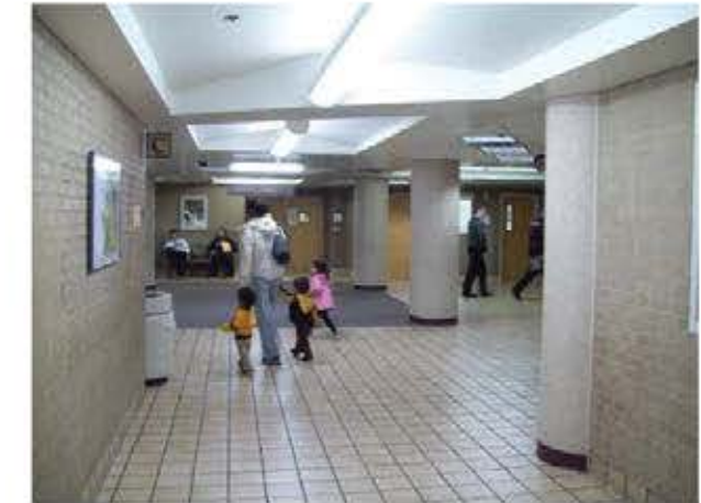
Lobby area, limited visibility to elevators
