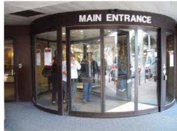
Main Entrance Revolving Door
