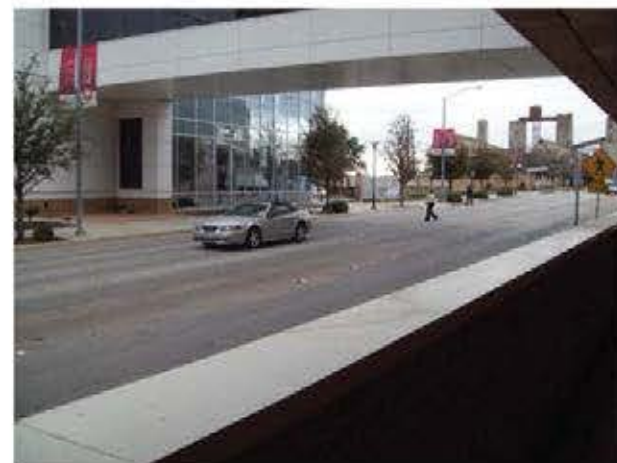
Main Street separation between Pavilion and Main Hospital
